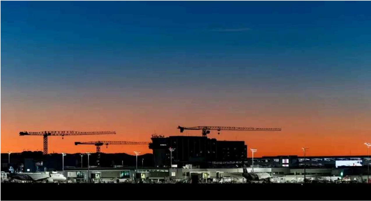
Auckland Airport construction.
